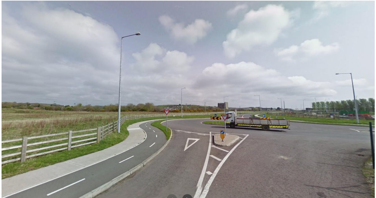
Figure 2.3 Existing Local Road lighting
