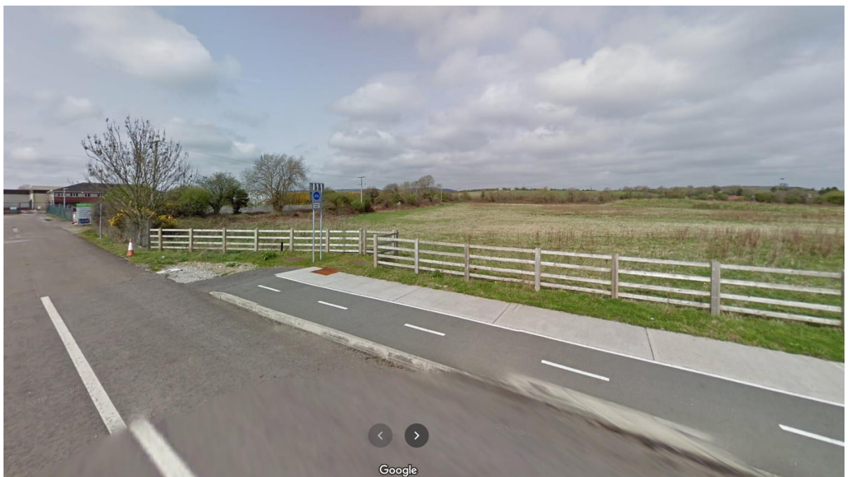
Figure 2.4 Existing Local Road lighting/ Development entrance location
