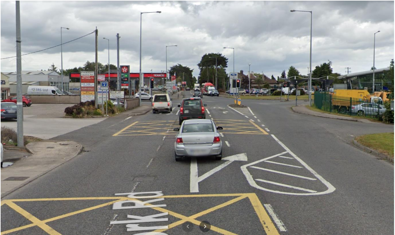
Figure 14.11 Eastbound (Credit: Google)
