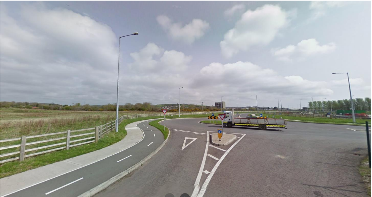
Figure 14.3 Eastbound (Credit: Google)
